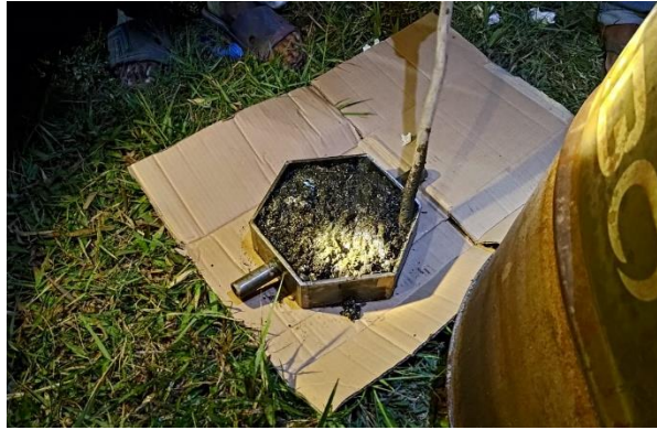
Gambar Proses Pencetakan Bata beton ( paving block )
